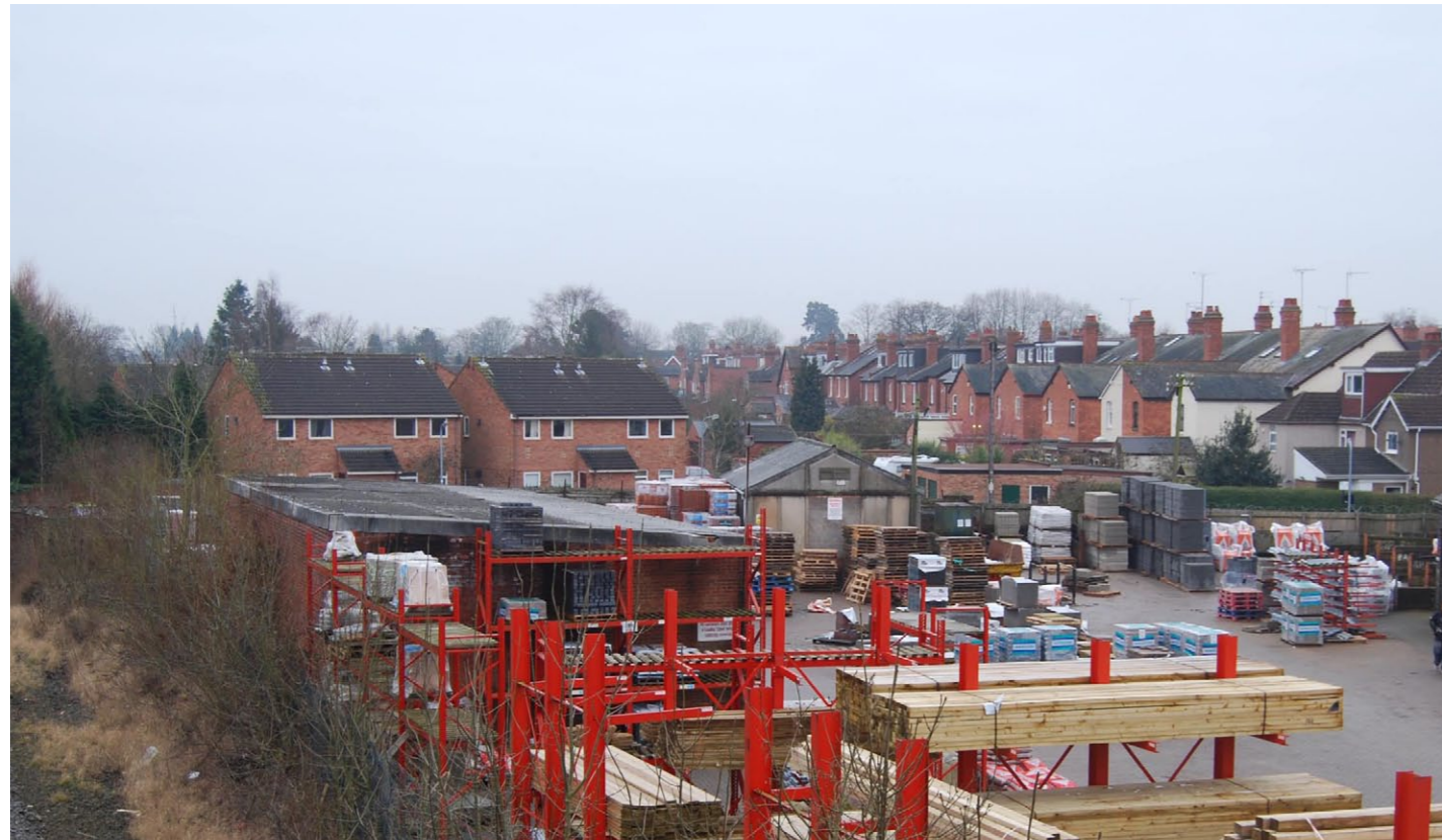
View of existing Yard from Footbridge
